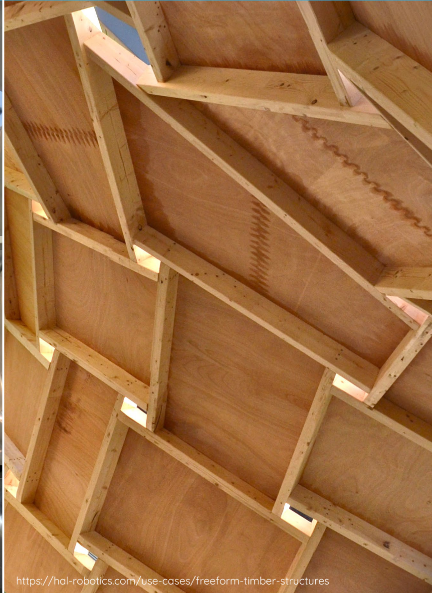
multi-robot prefabrication of doubly-curved timber shell Construire le Courbe, ENPC build'in et al.
